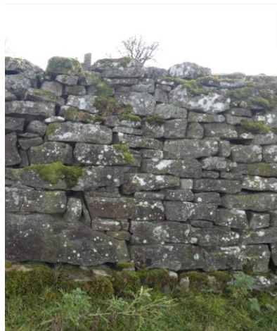
Fig. 8 A length of wall with straight sides, flat topstones, a plinth and a blocky nature
