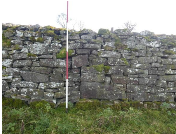
Fig. 9 The straight joint in the dividing wall, right of the ranging pole, showing the difference in stone type and characteristics either side
