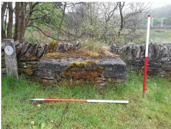
Figure 17 Churn stand (J076) located on the former Lunes Bridge.
