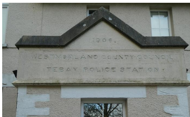
Figure 8 Date stone (J054) of 1906 on the former Police Station.
