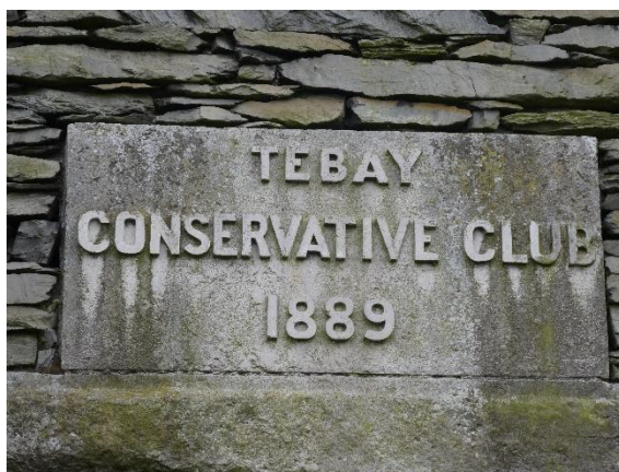
Figure 7 Date stone (J074) of 1889 on the former Conservative Club.
