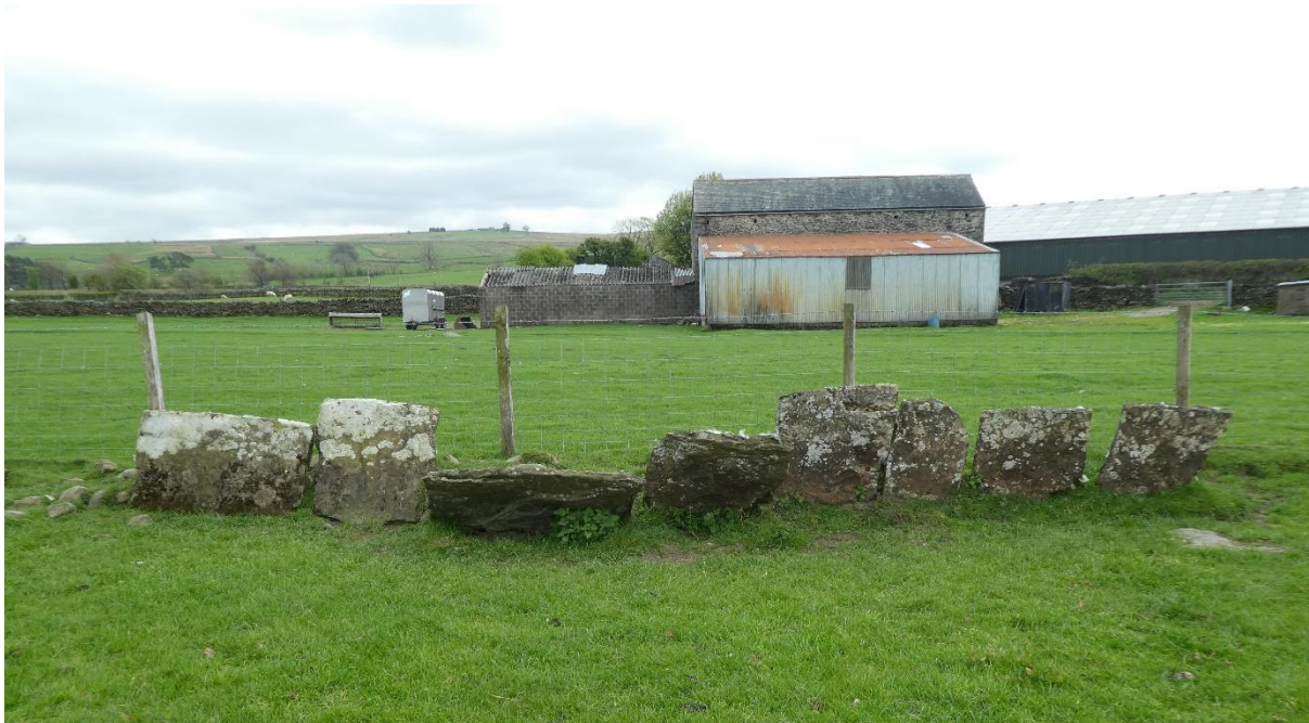
Figure 19 Vertical slab wall (J064) situated in a field on the outskirts of Old Tebay.
