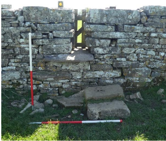
Figure 20 West side of step stile A072 - with two freestanding steps, which are possibly replacing a broken throughstone.
