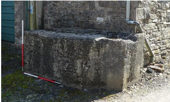
Figure 24 Churn stand (A040) is encased in concrete.
