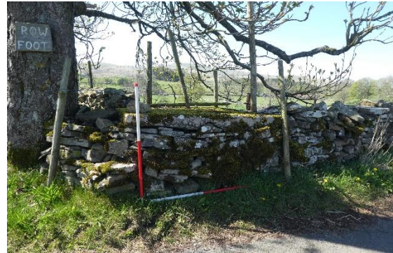
Figure 25 Churn stand (A074) is built into a dry stone wall.
