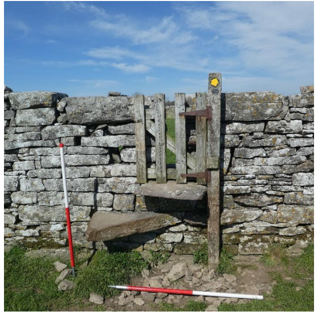
Figure 21 East side of A072 showing one protruding throughstone as step.
