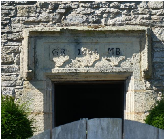
Figure 3 Date stone of 1604 (G088) on Petty Hall.
