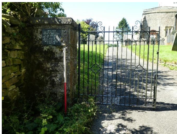
Figure 15 The plaques are attached to gate piers at the entrance to the churchyard.
