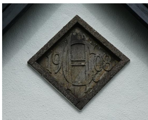
Figure 9 Date stone (G021) in a diamond shape with a frame that projects from the wall.
