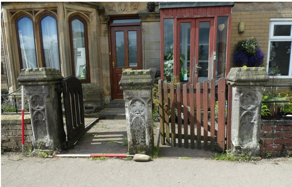
Figure 18 Gate piers (G009b) outside Swan Villa - the left and central pier lead to the original doorway, the one on the right appears to be a repurposed and relocated wall pier.
