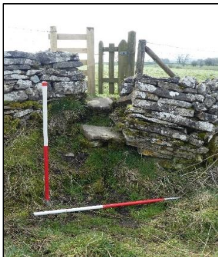
Figure 8: Image showing feature B05, a step stile with steps cut into the bank situated between the field and sunken lane.
