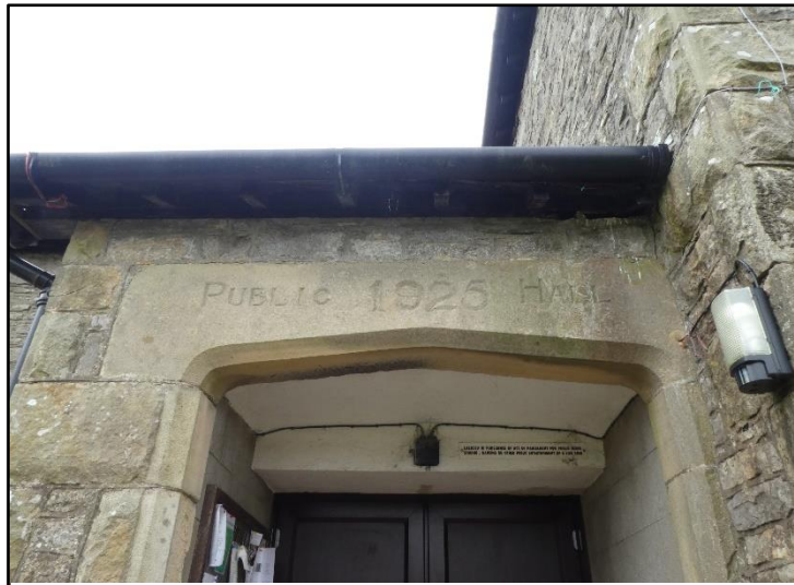
Figure 4: Image showing the inscribed lintel on the Public Hall in Newbiggin-On-Lune.
