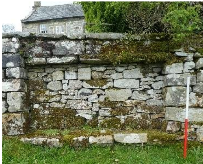
Figure 10: An unknown east-facing recess in the wall outside of Meaburn Hill (possibly a bee bole).
