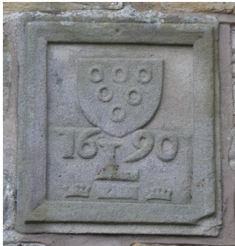
Figure 4: Image showing date stone. Lowther crest above the cart door on the old mill.
