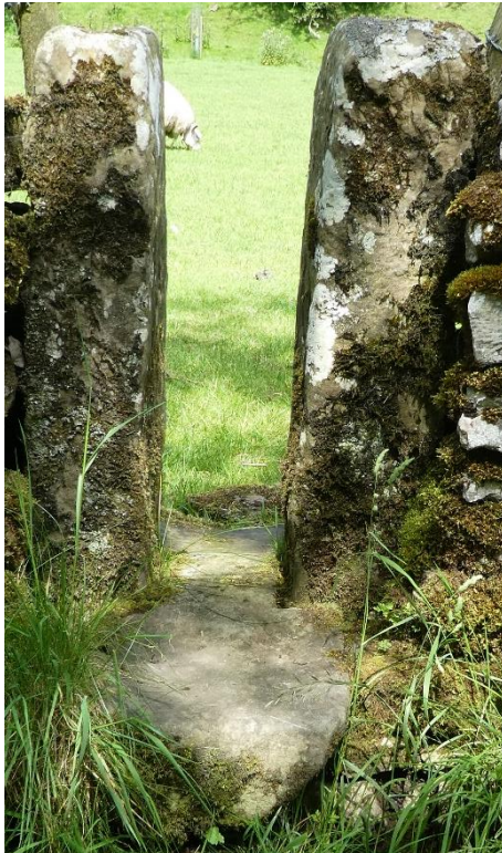
Figure 11: Left - Image showing how the horizontal stone has been shaped around the vertical stones of squeeze stile E013. Right – Image showing the squeeze stile E011a built into the wall with a gate stoop (E011a) on the right.
