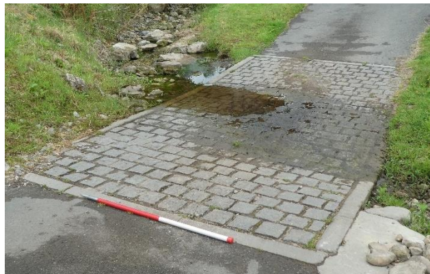
Figure 11: Ford to the south of the village (C071) showing the modern stone-sets and curbing.
