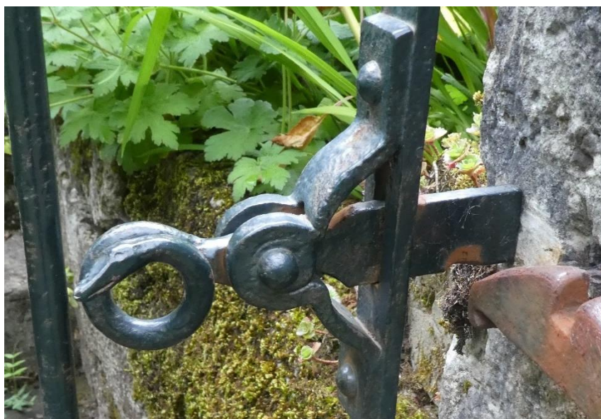
Figure 16: Image showing the gate latch on the gate between a pair of gate stoops (C076).
