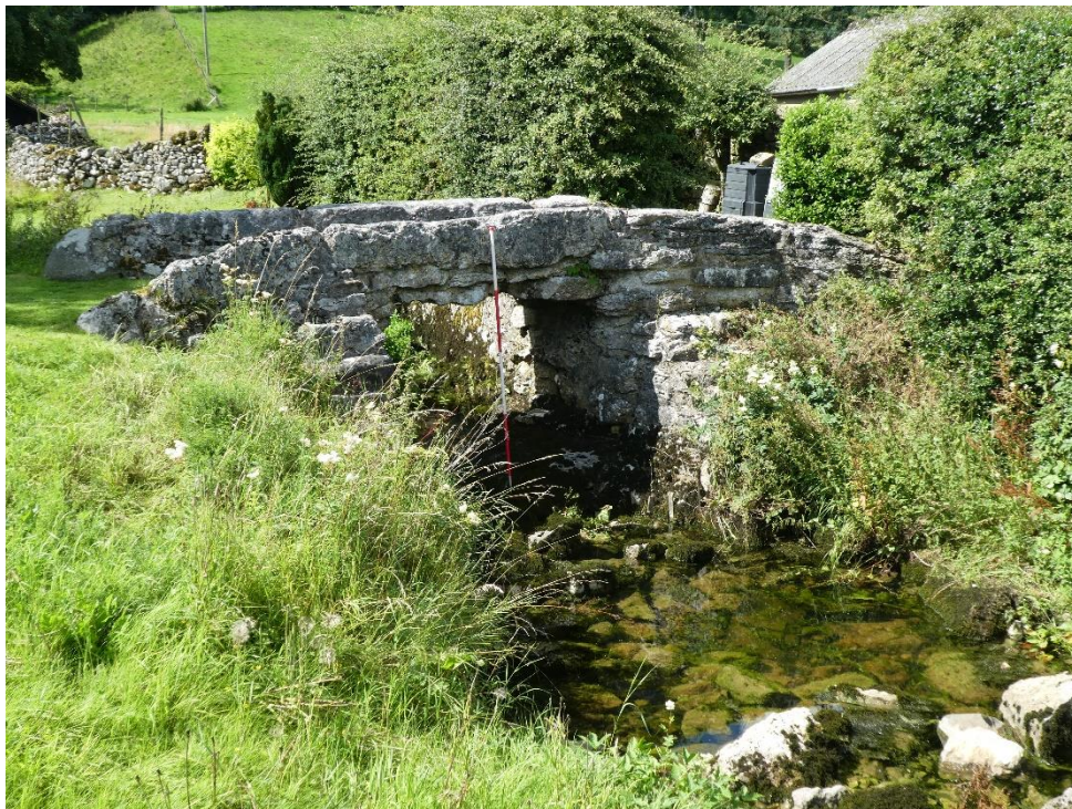
Figure 17 Footbridge crossing Dale Beck (D216)
