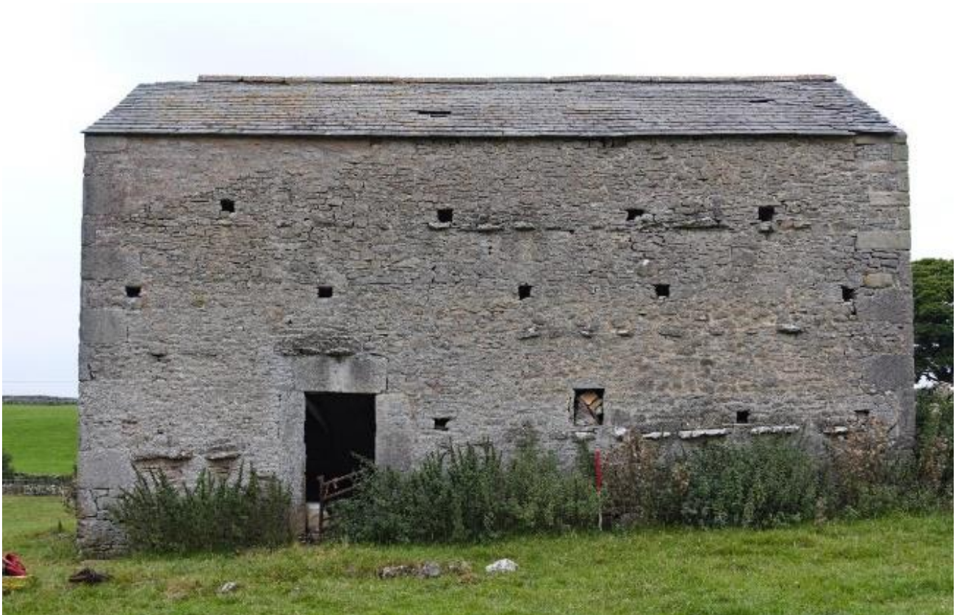
Figure 5 A field barn surveyed in the Westmorland Dales.
