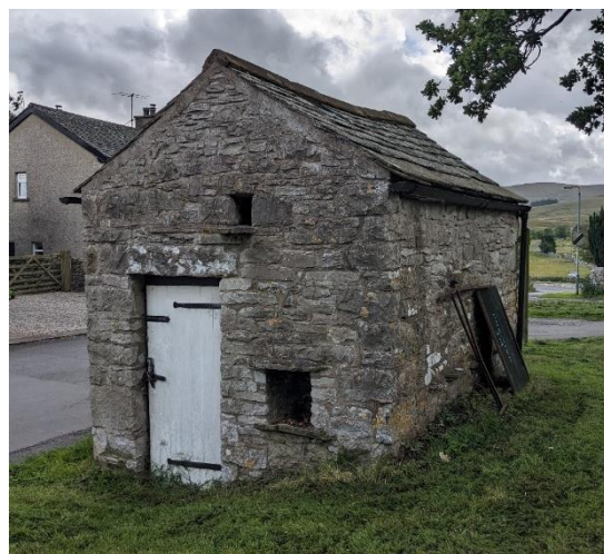
Figure 4 Hennery-piggery located on green space at the south end of Ravenstonedale (not surveyed). It has the characteristic chute for pig-feed and small loft opening for hen access.
