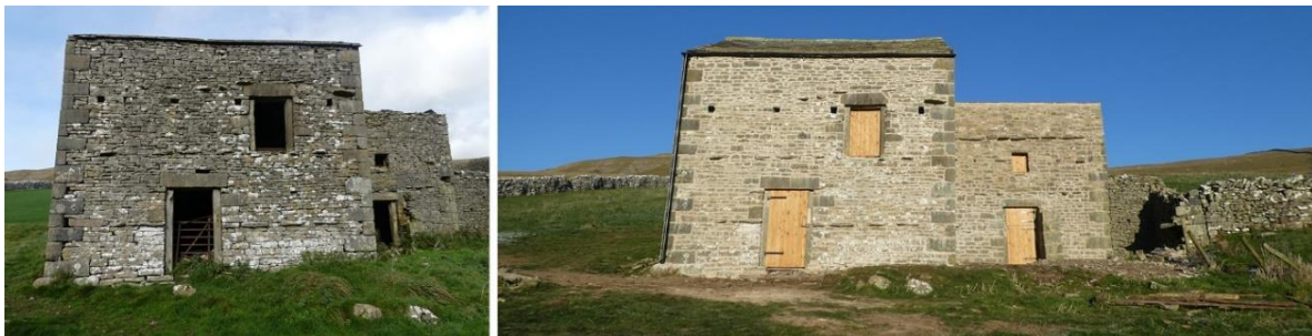
Figure 1 Bank barn situated on the coast-to-coast - before repairs (left), after repairs (right).
