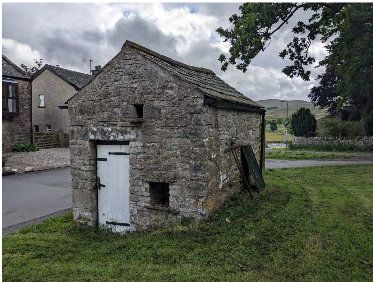
Figure 38 Hennery-piggery located on green space at the south end of Ravenstonedale (not surveyed). It has the characteristic chute for pig-feed and small loft opening for hen access.
