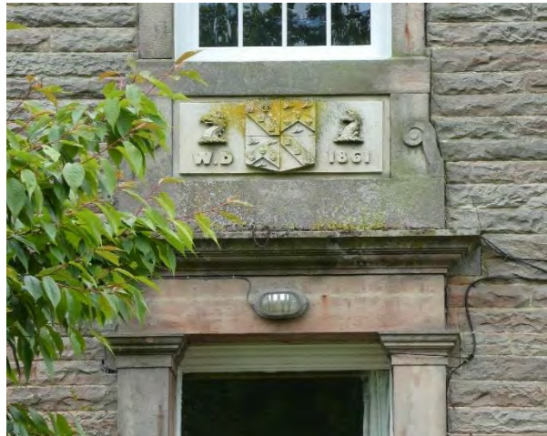
Figure 65 1861 datestone located on front elevation of Midtown Farm.
