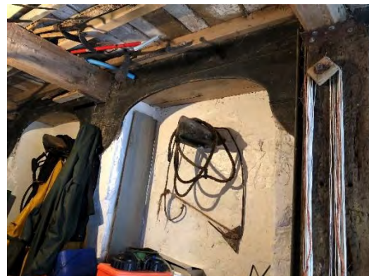
Figure 47 Evidence of brackets to hold small harness saddles or pads.
