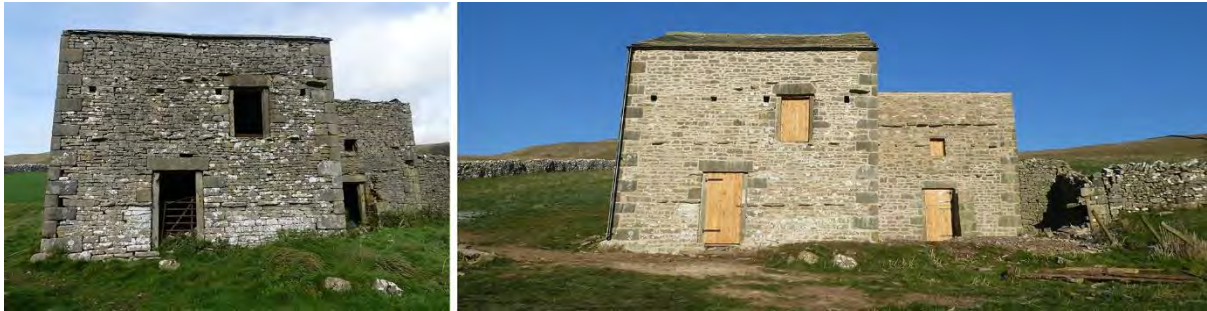
Figure 80 Bank barn situated on the coast-to-coast - before repairs (left), after repairs (right).
