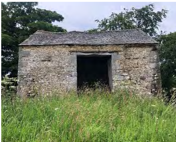
Figure 27 First floor of field barn accessed by bank (Crosby Ravensworth parish).
