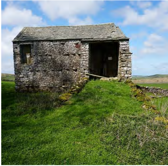
Figure 29 First floor of field barn accessed by constructed ramp (Asby parish).
