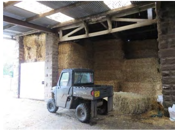
Figure 57 One of the pillars has been removed from this open elevation.
