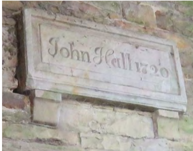
Figure 60 Reused datestone on the farmstead.
