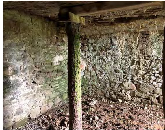
Figure 22 Interior of turnip store located under ramp.
