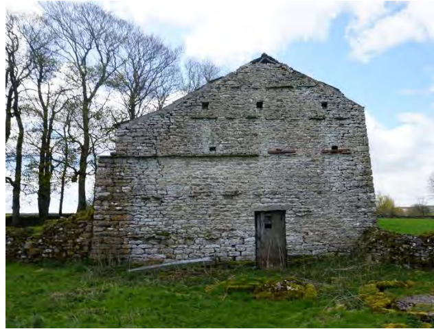
Figure 30 Ground floor access into the byre, with revetment for constructed ramp visible to left.
