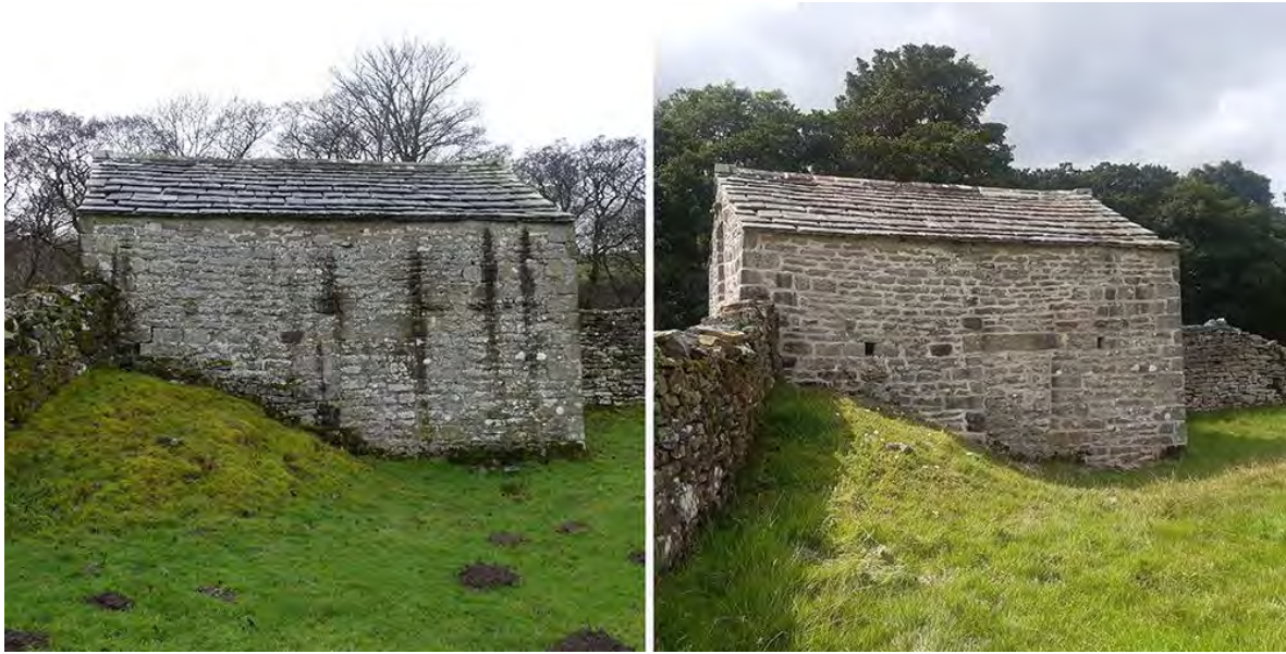
Figure 78 Field barn on the site of Pendragon Castle - before repairs (left), after repairs (right).
