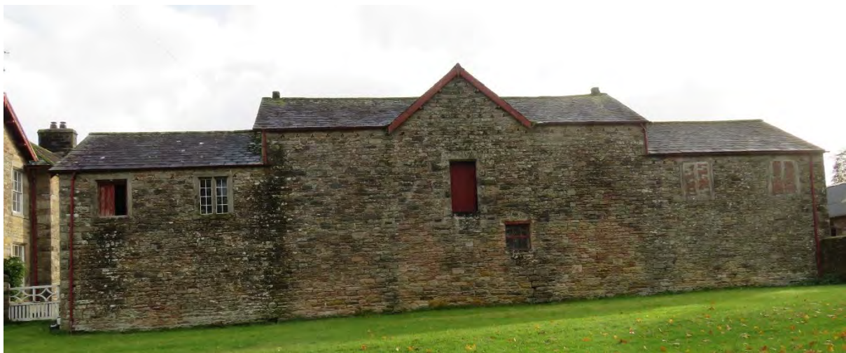
Figure 59 West-facing (roadside) elevation as it appears today.
