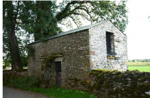
Figure 32 Field barn, located on roadside (Ravenstonedale parish).
