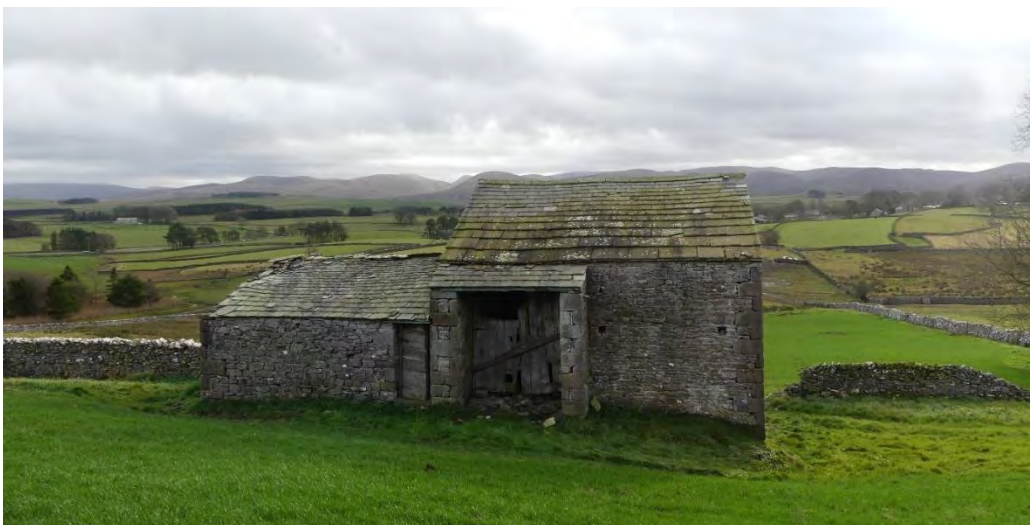
Figure 81 The north-facing elevation with cart entry (photo taken pre-repair works).
