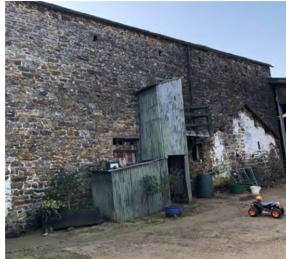
Figure 40 Corrugated iron chute.
