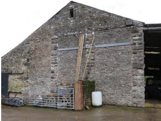
Figure 56 Gable end, which was originally open, has been filled in.
