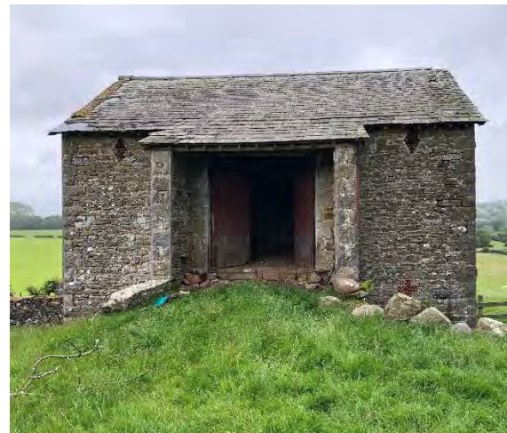
Figure 24 First floor access to bank barn, accessed by ramp.
