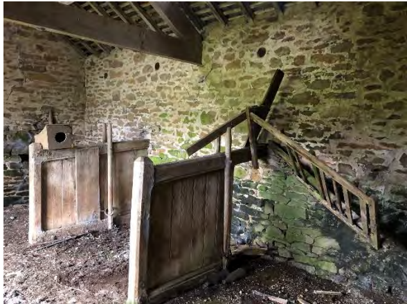
Figure 45 Interior of single-storey byre with wooden boskins and rudsters surviving.
