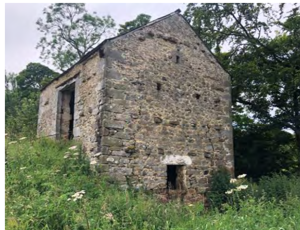
Figure 28 Ground floor access into the byre. Former roofline shows that this barn has been heightened.
