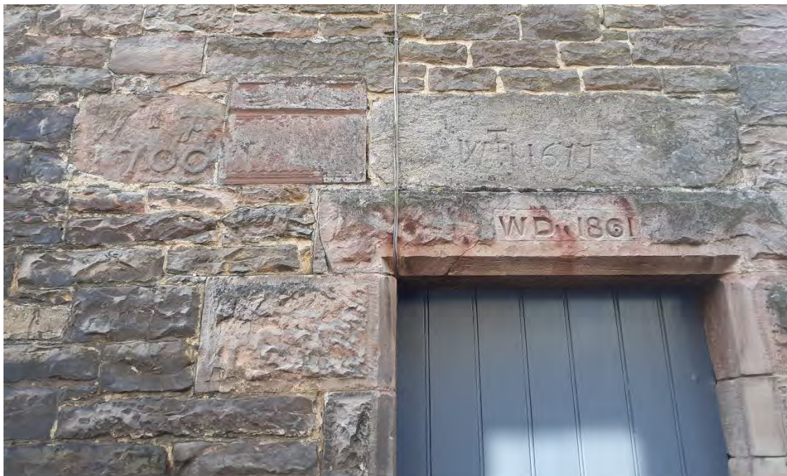
Figure 71 Gable end with a number of datestones - reused datestones of 1677 and 1700 with the initials 'W T H' and a datestone for the rebuild of 'WD 1861'.
