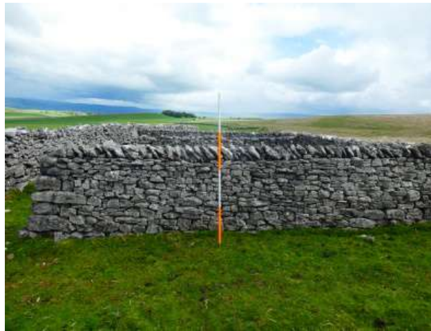
Fig. 66 Wall no. 10, sheepfold, looking east through the two cells (2m scale)
