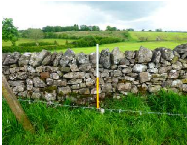
Fig. 58 Wall no. 24, an enclosure wall of 1849, looking south-west (1m scale)
