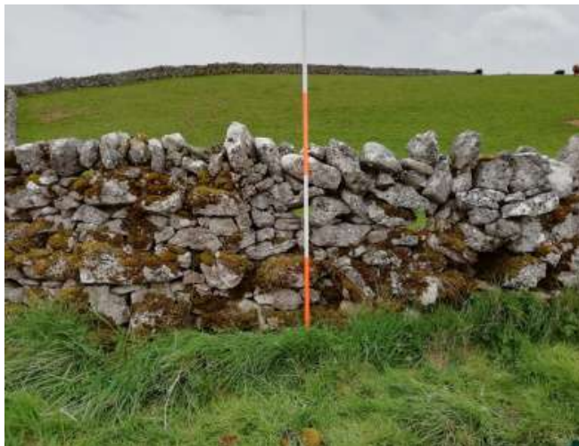
Fig. 56 Wall no. 4, an enclosure wall of variable build-quality, looking north (2m scale) (Steve Blenkinsop)
