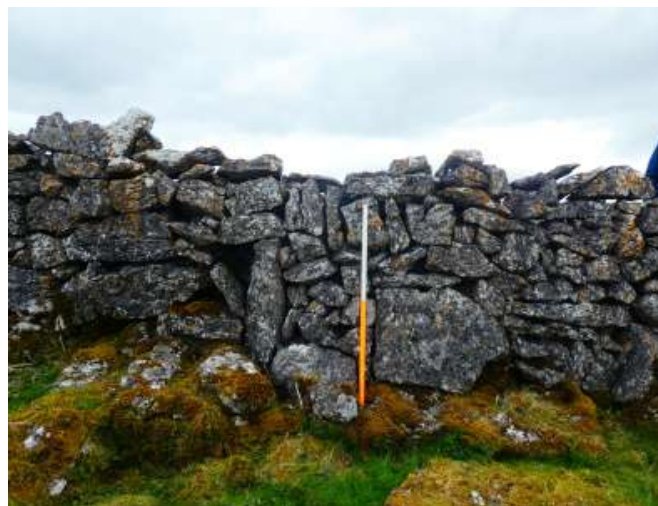
Fig. 44 Wall no. 6 looking west. The join between one phase and another is seen just left of the (1m) scale
