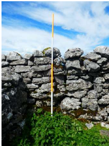
Fig. 79 Wall no. 9, a blocked-up squeeze stile within a sheepfold at NY68769 10087 (2m scale)
