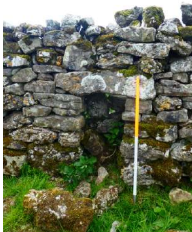
Fig. 76 Wall no. 27, a tall and narrow sheep creep (1m scale)
