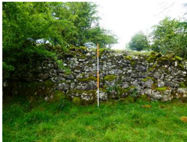
Fig. 53 Wall no. 37 showing its height and 'crude' nature looking south (2m scale)
