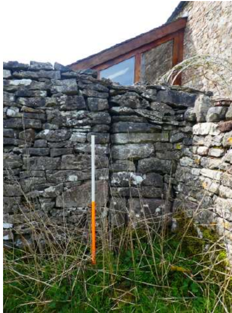
Fig. 74 Wall no. 18, showing a clear straight joint (1m scale)
