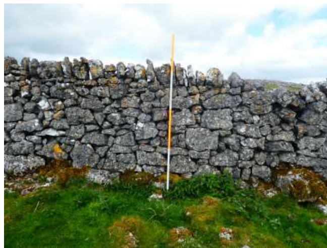
Fig. 42 Wall no. 5 showing the lack of coursing, looking west (2m scale)
