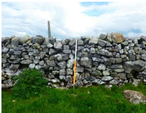
Fig. 59 Wall no. 27, an enclosure wall of 1855, north (1m scale)
