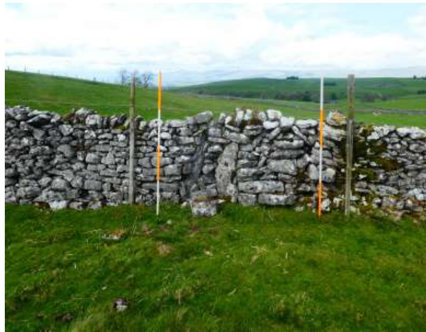
Fig. 77 Wall no. 9, a blocked cattle creep at NY68462 10028 (2m scales)
