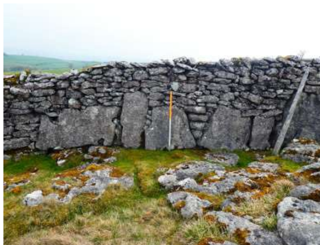
Fig. 29 Wall no. 8, showing the earlier orthostat wall with later walling above, looking east (1m scale)
