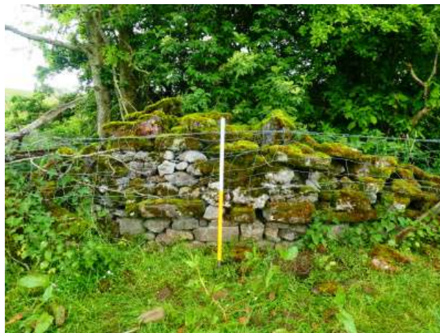
Fig. 52 Wall no. 32 showing its blocky nature, looking south-west (1m scale)
