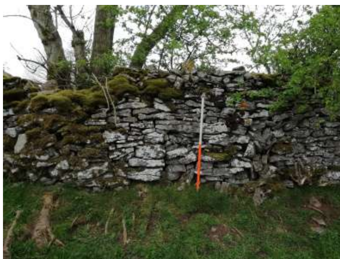
Fig. 40 Wall no. 1 showing its crude nature, straight sides and flat top looking south-west (1m scale) (Steve Blenkinsop)
