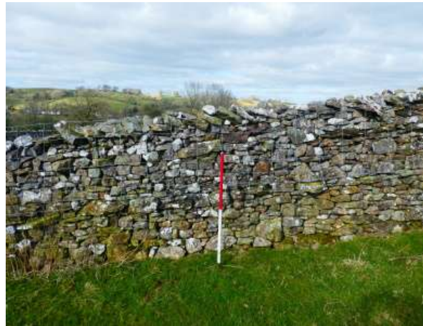
Fig. 69 Wall no. 21 showing its mixed geology, looking north (1m scale)
