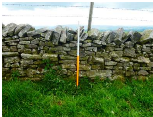
Fig. 61 Wall no. 29, the northern section, looking north-east (1m scale)
