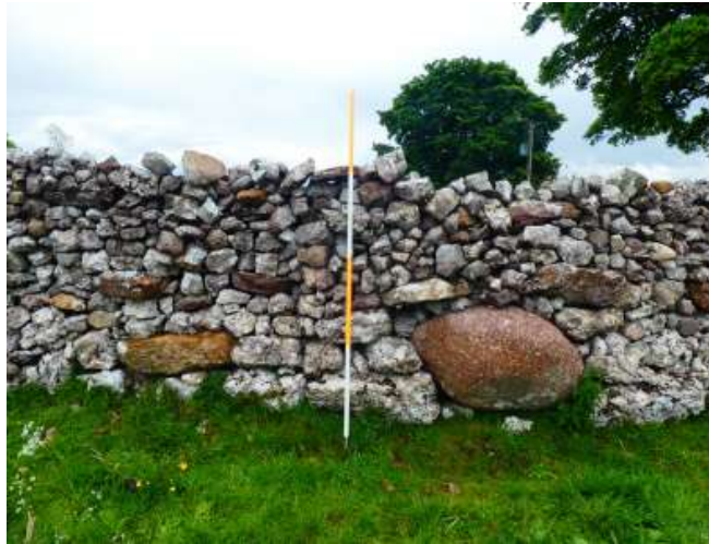
Fig. 50 Wall no. 23 with numerous Shap Granite erratics and a plinth at the base, looking north-east (2m scale)
