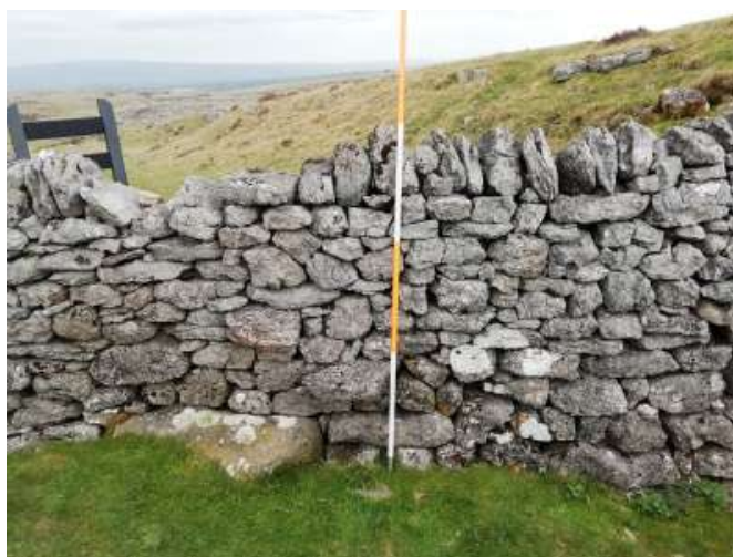
Fig. 41 Wall no. 2 with a Shap Granite basal slab visible, looking east (2m scale) (Steve Blenkinsop)
