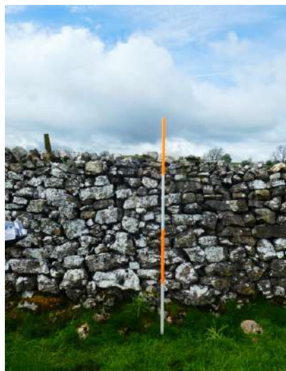
Fig. 48 Wall no. 14 showing its flat top and lack of coursing looking west (2m scale)
