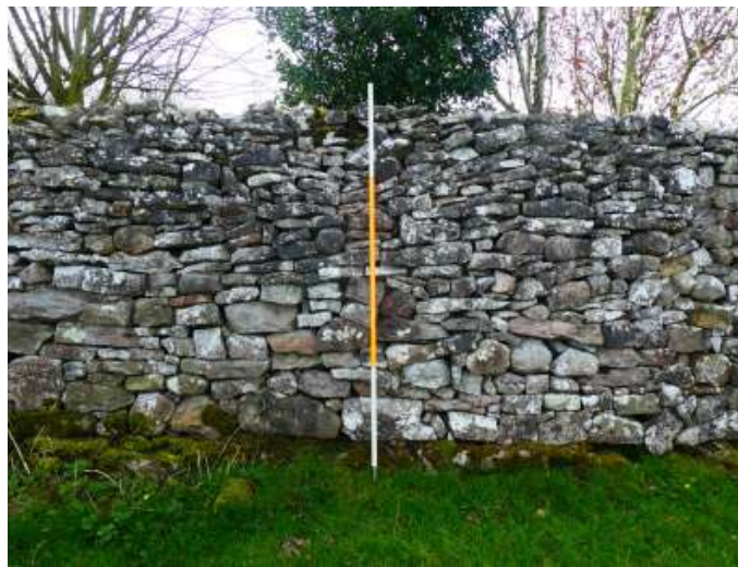
Fig. 49 Wall no. 18 showing its flat top and partly blocky nature, looking west (2m scale)
