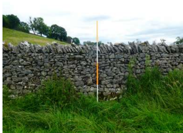
Fig. 71 Wall no. 34, looking north-east (2m scale)
