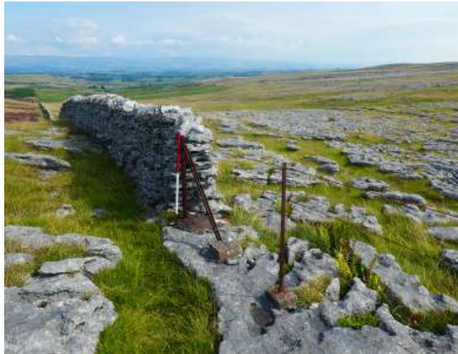
Fig. 55 Wall no. 3 replaced by post-and-wire fencing
