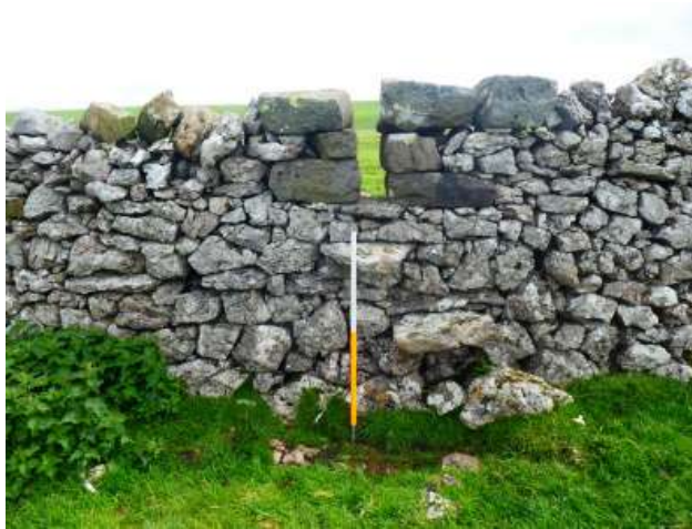
Fig. 78 Wall no. 13, a step stile with modern additions at the top (1m scale)
