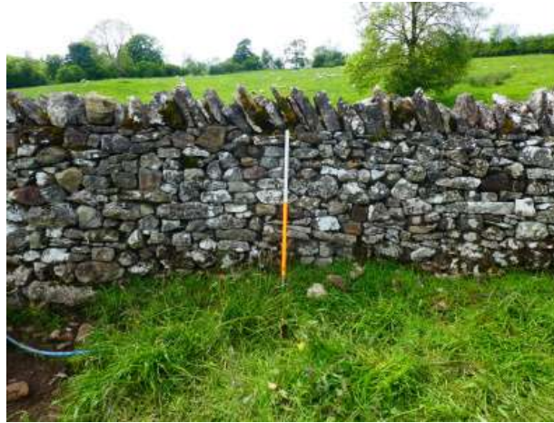
Fig. 70 Wall no. 31 looking north (1m scale)
