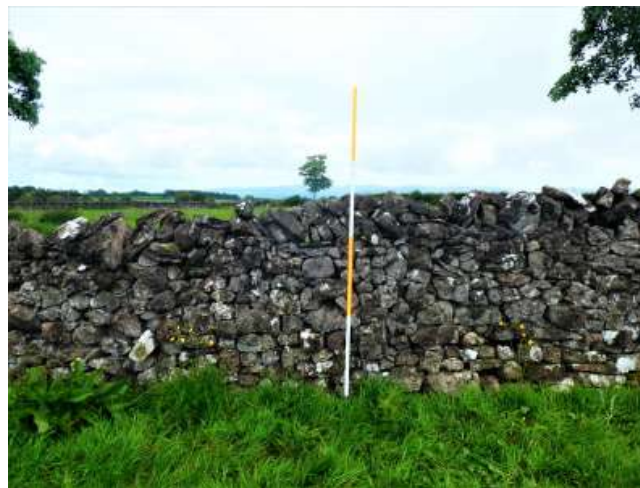
Fig. 57 Wall no. 22, an enclosure wall of 1849, looking south-west (2m scale)
