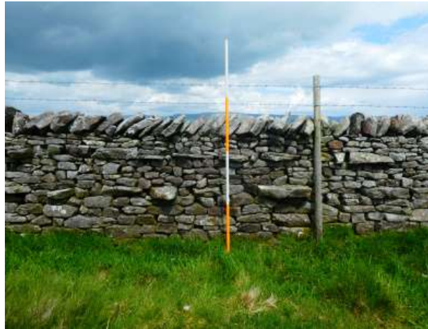
Fig. 62 Wall no. 29, the southern section, looking north-east (2m scale)
