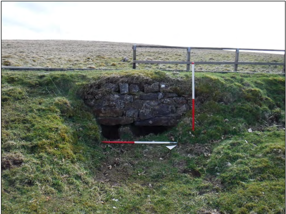
Plate 45: south side of the revetment and culvert M422.
