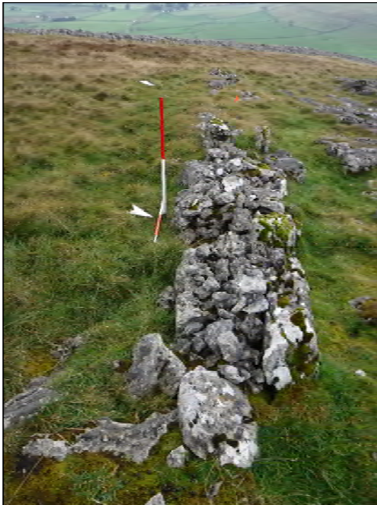
Plate 39: (right) wall D53 looking south down the length of the wall. The wall is formed of large stones on the exterior of the wall with rubble infill.
