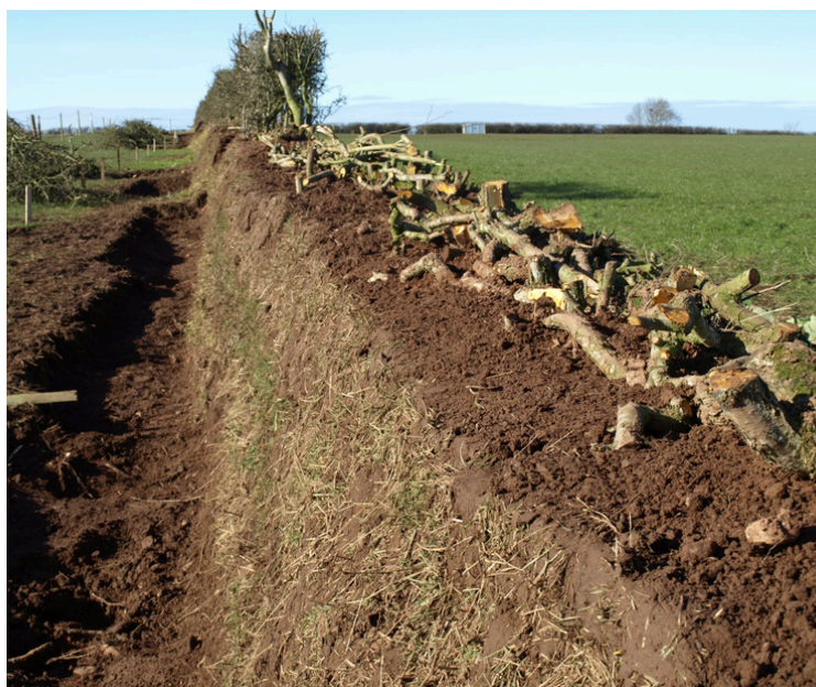
Above: A restored earth bank on the Solway, tall to protect the hedge roots against frequent flooding
